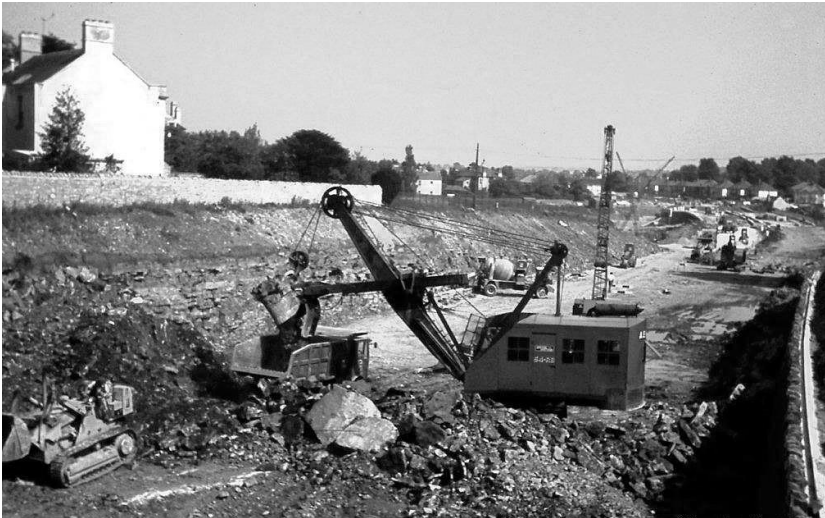
Station Road Cutting with a Ruston Bucyrus 54RB Face Shovel loading a Scammel Dump truck. Garth Reed operated the 54RB
